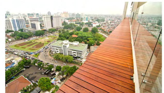
Softline Merbau Decking - Jakarta
