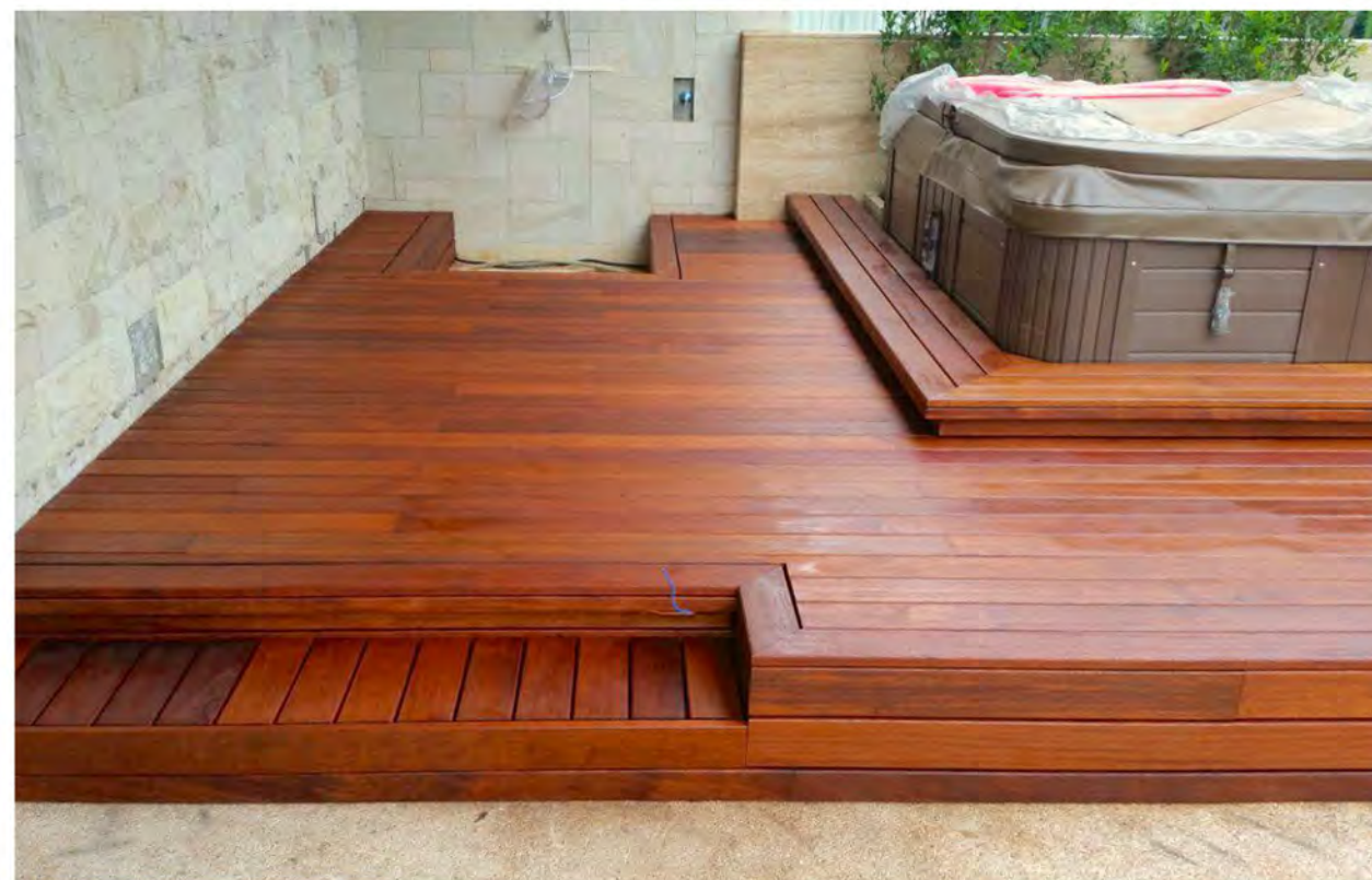
Softline Merbau Decking - Jakarta
