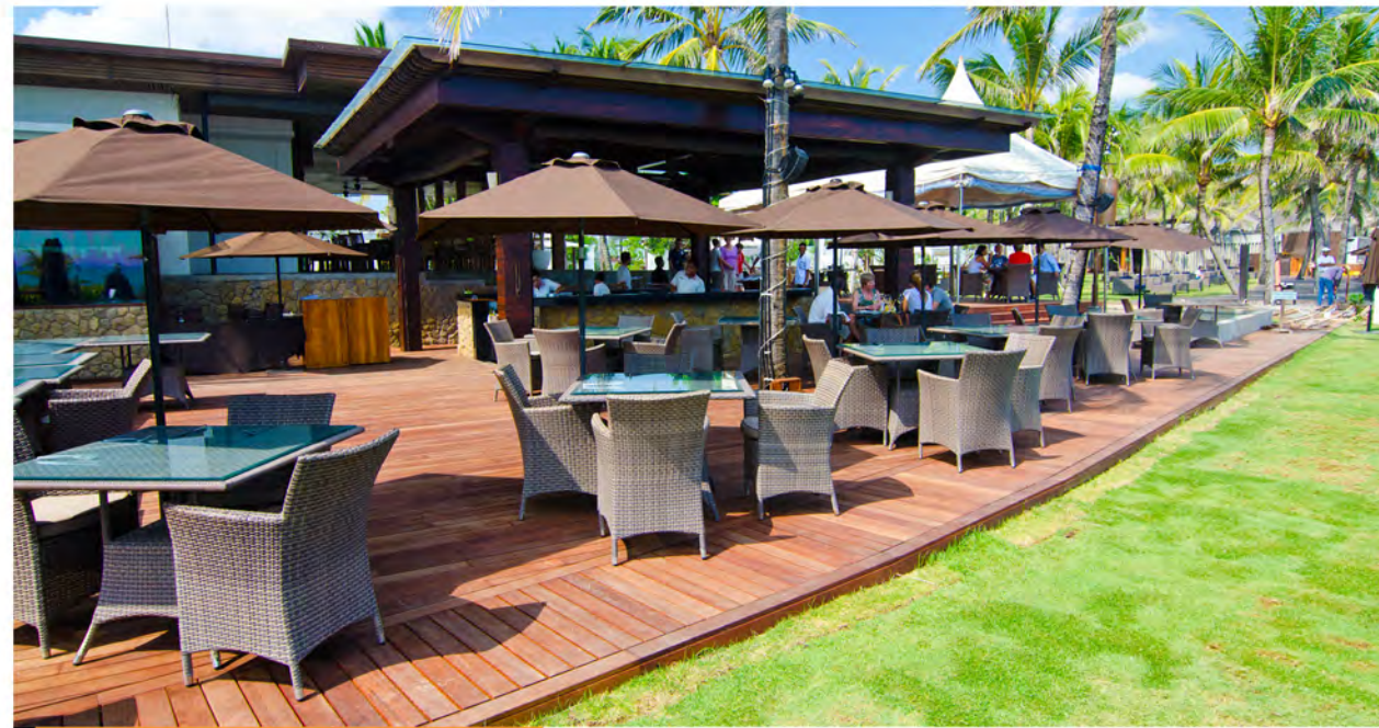
Softline Merbau Decking - Samaya Resto & Villa, Bali
